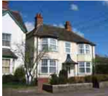
D - A345, Amesbury Relevant design elements: - symmetrical elevations - render - detached house - hipped roof - low boundary wall
