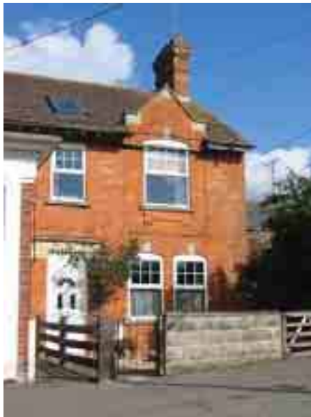
C - Bulford Road, Durrington Relevant design elements: - accomodation in roof space - brick elevations - chimney
